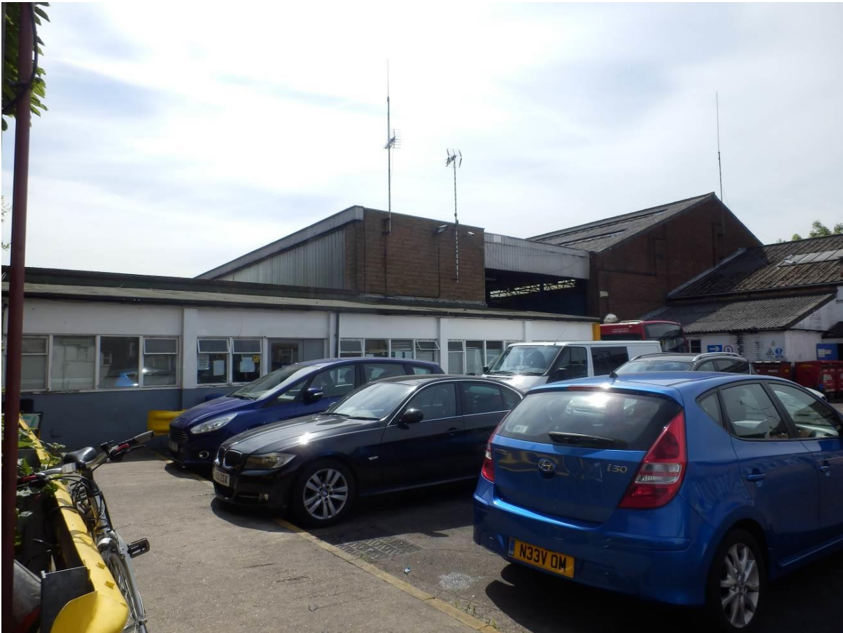
Larger service building, and additional buildings behind Marlow Court to be demolished
