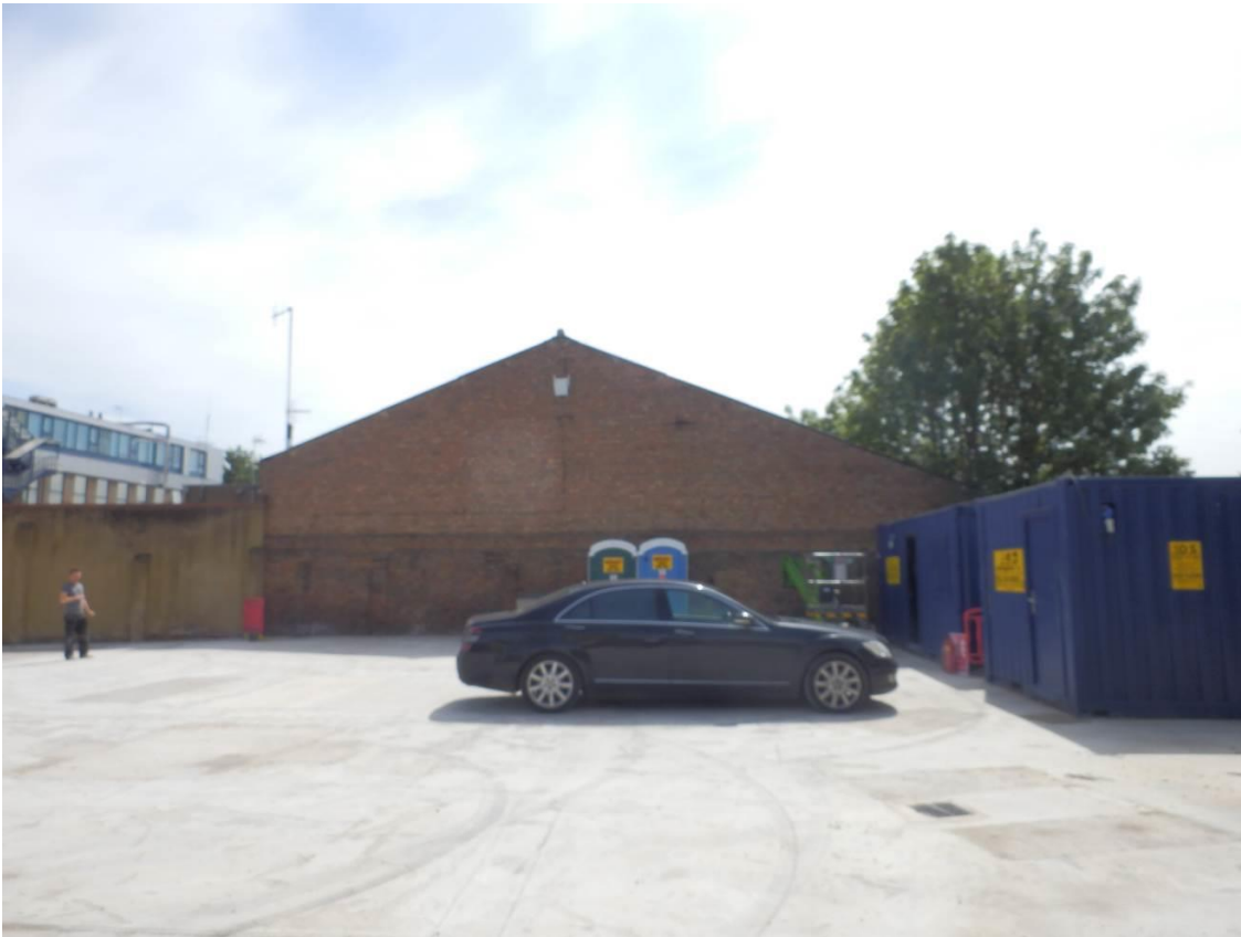
Looking towards existing bus depot buildings
